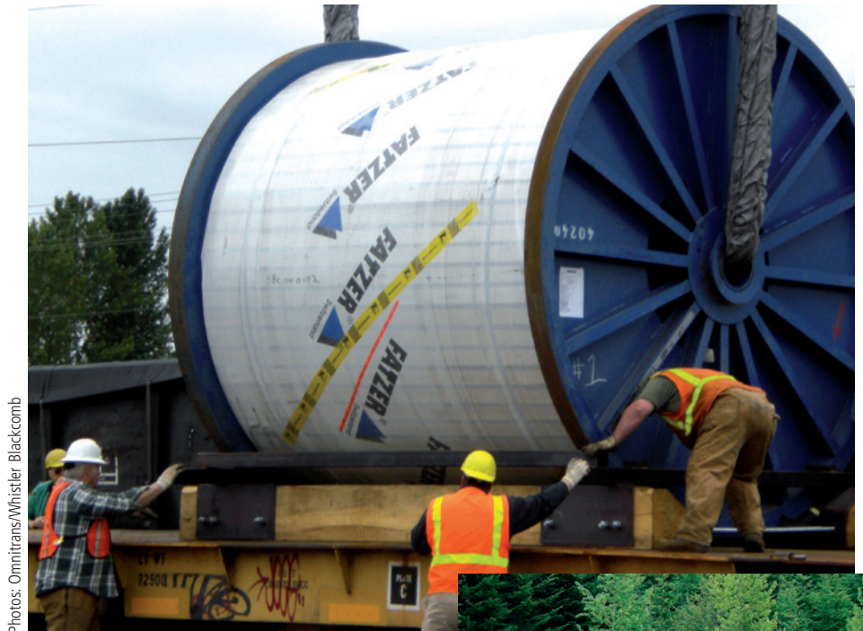
Coils of steel rope on their way to the construction site of a record-breaking aerial tramway in Whistler Mountain (Canada).
